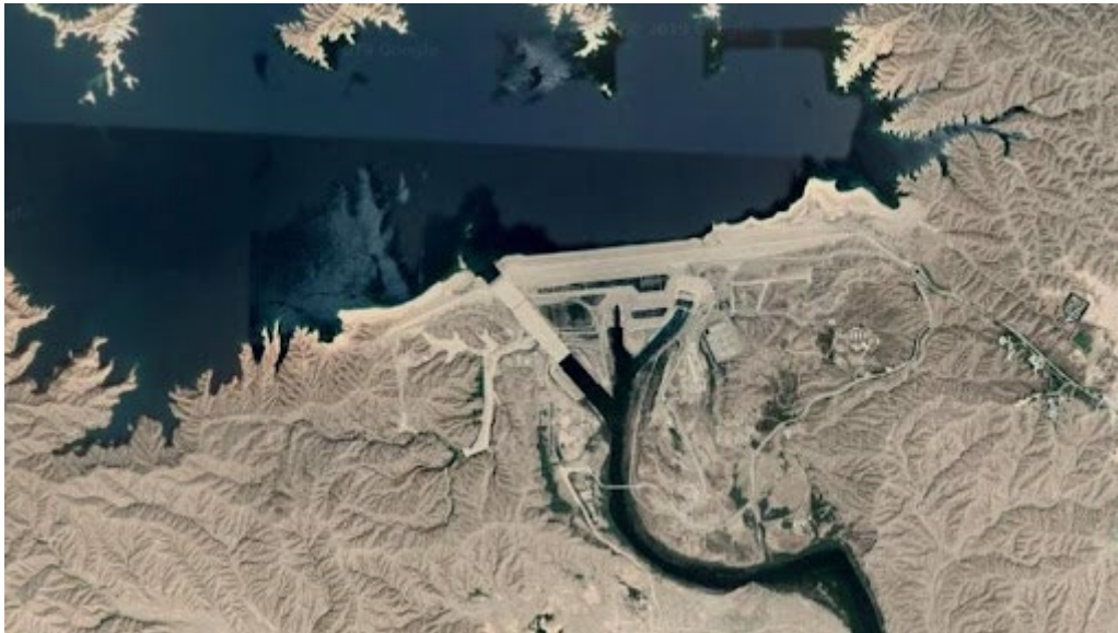
Figure 2. Karkheh embankment dam (Google Earth).
